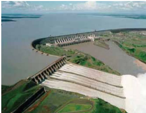
Figure 7. Itaipu Dam, located at the Paraná River on the border between Brazil and Paraguay. The Itaipu's reservoir is the seventh largest in Brazil, but has the best relation between electricity production and flooded area – see Table 1. Source: www.itaipu.gov.br
