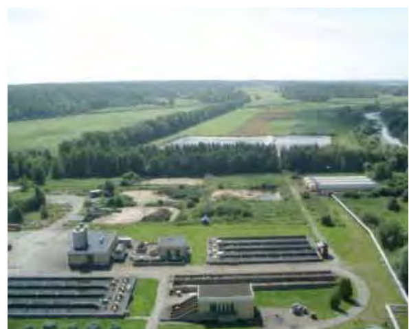
Figure 31. View of municipal wastewater plant, with water storage ponds and (behind the ponds) willow fields that are used as vegetation filters for the treatment of pre-treated municipal wastewater. The photo is taken from the roof of the heat and power plant that uses the locally produced biomass. Courtesy: Pär Aronsson, Swedish Agriculture University.
