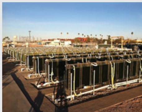
Arizona State University Algae Testbed Public-Private Partnership flat-panel photobioreactor
